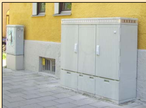
Figure 6 Mobile base-station, normal distribution cabinet and UCV
